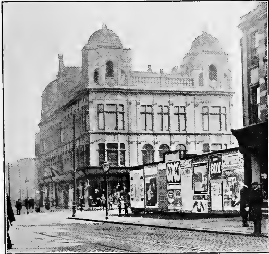
SLIDE No. 100.—THE PROPOSED GARDENS WOULD BE OF ENORMOUS ADVANTAGE TO THIS BUILDING.
